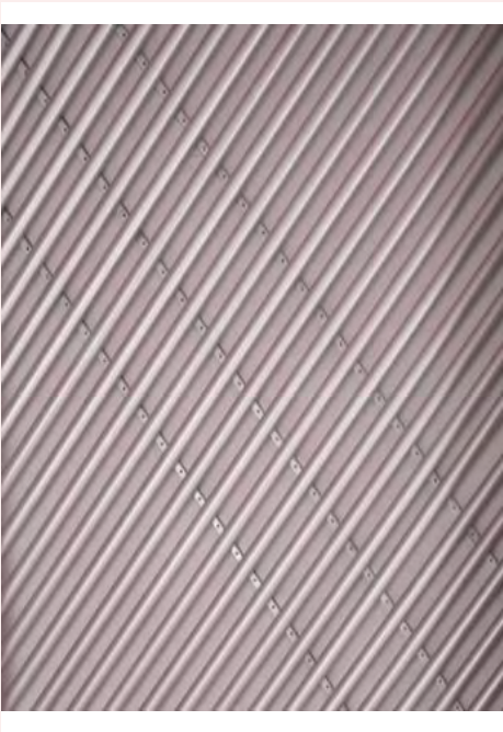
Installed Ø 50 mm tubes
