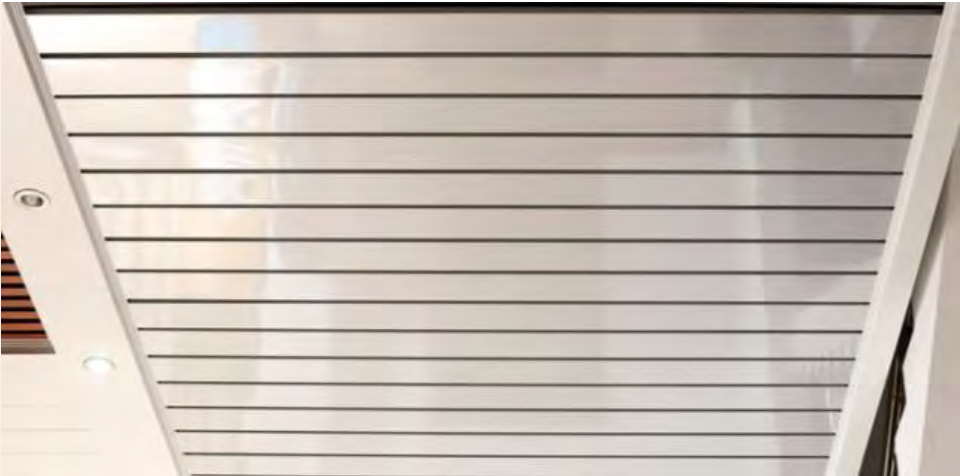
Installed H-profile ceiling
